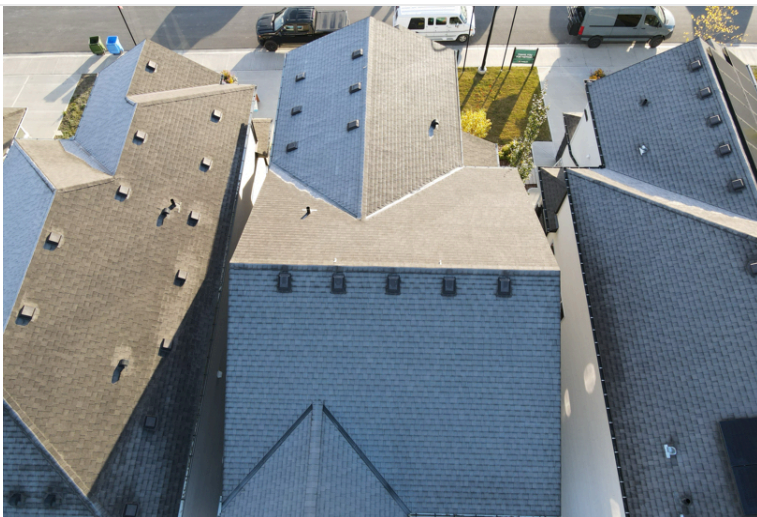
Roof Back View
