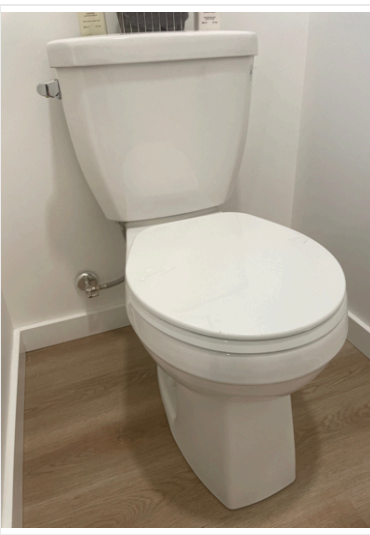
Thermal Toilet Scanned for leaks at the base, tank & shut-off valve.
