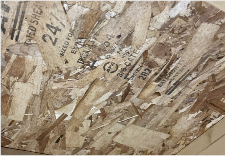
Attic Sheathing "Roof Sheathing" Here are the boards or sheets that bridge the trusses or rafters.
