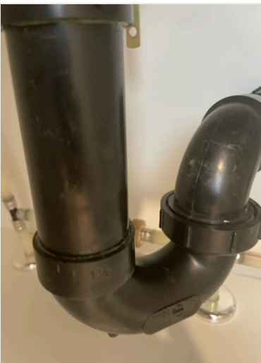
Thermal P-Trap Scanned for leaks or the presence of moisture.
