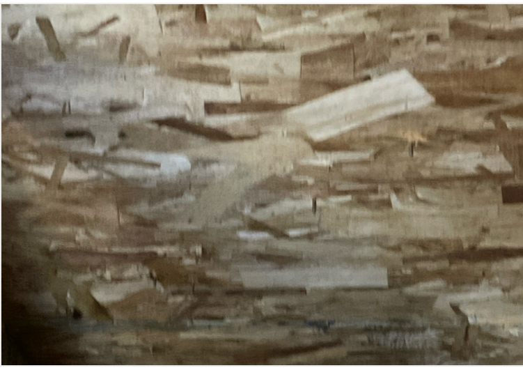
Roof Sheathing The thin boards of wood that span the trusses and support the rest of the roof
