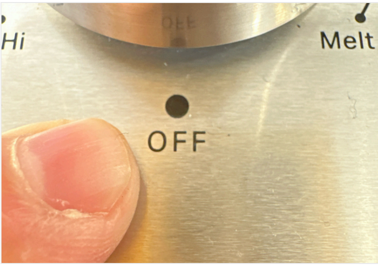
Stove • Oven Off Turned ON & OFF after testing for functionality.
