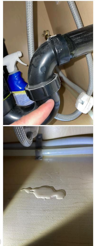
• **Basement Bar Sink P-Trap** P-traps are part of your sink plumbing, these question-mark-shaped plumbing pieces serve an important purpose... Active Leak. Repair or Replace.
