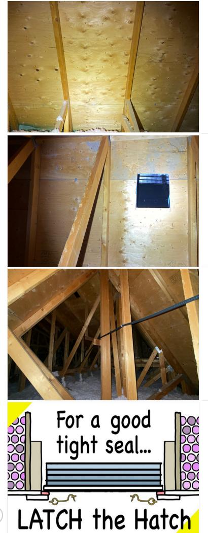
**Roof Sheathing** The thin boards of wood that span the trusses and support the rest of the roof
