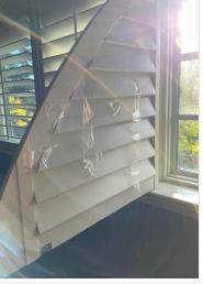
• **Shutters** A type of air opening, usually covered by one or more moving flaps. Damaged. Repair or Replace.
