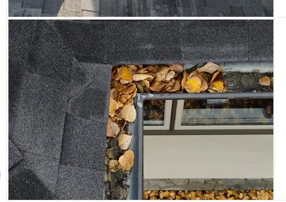
• Inside Gutter Responsible for channeling water flow from your roof through the downspouts & direct it to appropriate areas. Regular cleaning of trough/scupper should be part of your yearly maintenance schedule. Debris Filled. Service Advised.
