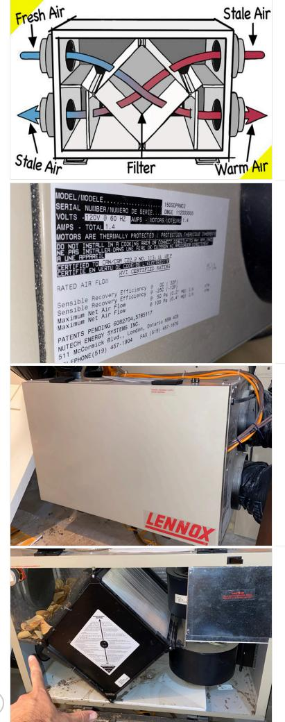
**HRV** Heat Recovery Ventilators exchanges indoor and outdoor air, using heat from outgoing air to warm incoming fresh air, optimizing energy use and improving indoor air quality. Excellent at reducing heating costs and preventing moisture buildup.
