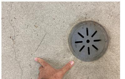
• Garage Floor Visually inspected for cracking, delamination, honeycombing & other common issues. Keep'er clean & free of debris. Minor Epoxy Deterioration. Monitor/Maintain.
