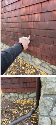
• Wood Siding Visually examined for common defects / For your records. Wood siding requires regular maintenance to preserve its appearance and struc Damaged. Repair or Replace.
