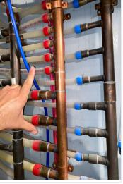
• Exterior Water Shutoff Valves These should be turned off & bled in the winter months to prevent potential problems in the spring. Missing Valve Handles. Replace.
