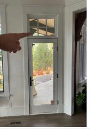
• Window Pane Visually examined for common defects. Cracked. Repair or Replace.
