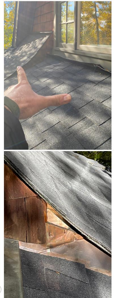
• **Roof Flashing/Cladding** Usually a thin metal material that is installed to direct water away from critical areas. Lifting/Missing. Repair.
