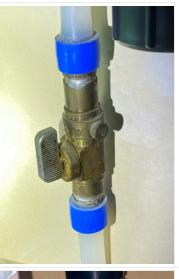
Main Water Shutoff Here in case of a leak! Also great when an appliance, mechanical or fixture needs to be replaced or serviced.
