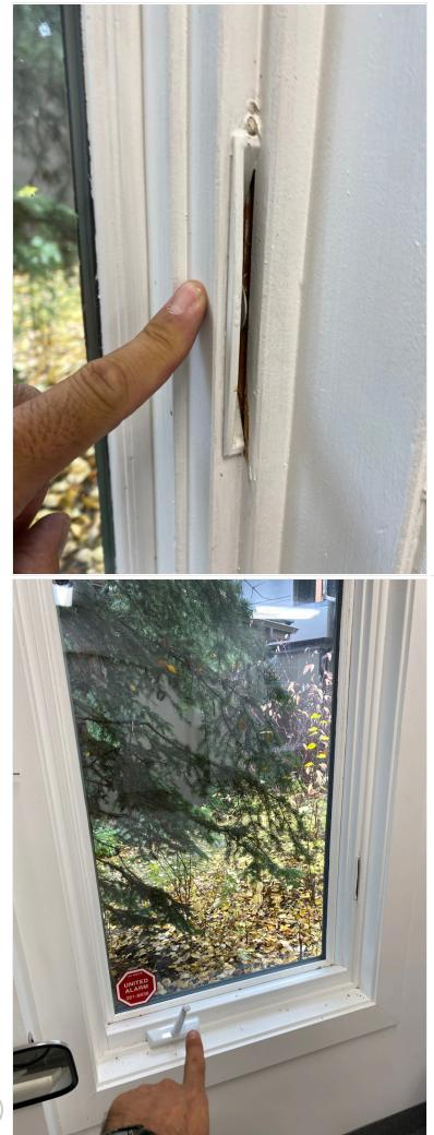
• Suite Garage Window These seem to be the primary way in for intruders. Video? Bars? Add some protection. Missing/Damaged Latch. Repair or Replace.
