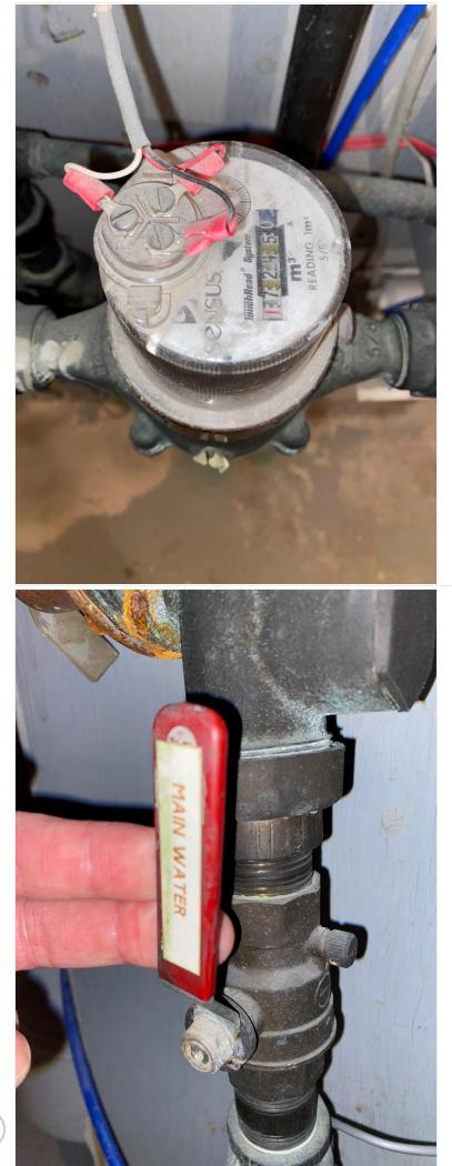
What does a water meter do? Water meters are essential in conserving water & saving money on your water utility statement. A water meter is a mechanical device connected to your water connection & only registers consumption when water is used. There are no electric components inside a water meter. Meters are usually installed just above the main water shutoff valve in the home & most water meters have a transmitter that is remotely read for billing purposes.
