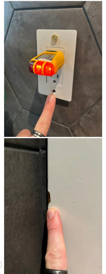
• Main Level Bathroom GFCI Note that GFCI reset is in upper shared bathroom Missing Screw. Replace.
