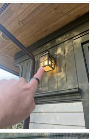
• **Light Fixture** Visually examined for common defects. Missing Components. Replace.
