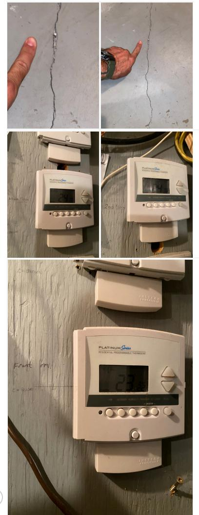
• **Basement Slab** Generally 4" thick, poured over 4" gravel & reinforcing wire. Crack(s). Seal/Monitor.
