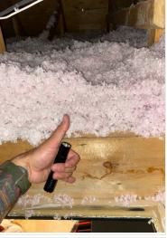
• Attic Hatch Skirt Also known as the hatch box. This type of surround is built as a sort of insulation STOP. To prevent insulation from falling on your fa Staining. Improve.
