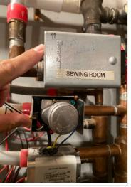
• Hydronic Zones: upper levels Entry/Mudroom thermostat was finicky & would not turn up high enough to test. Service system & confirm function. No Function. Further Evaluate.
