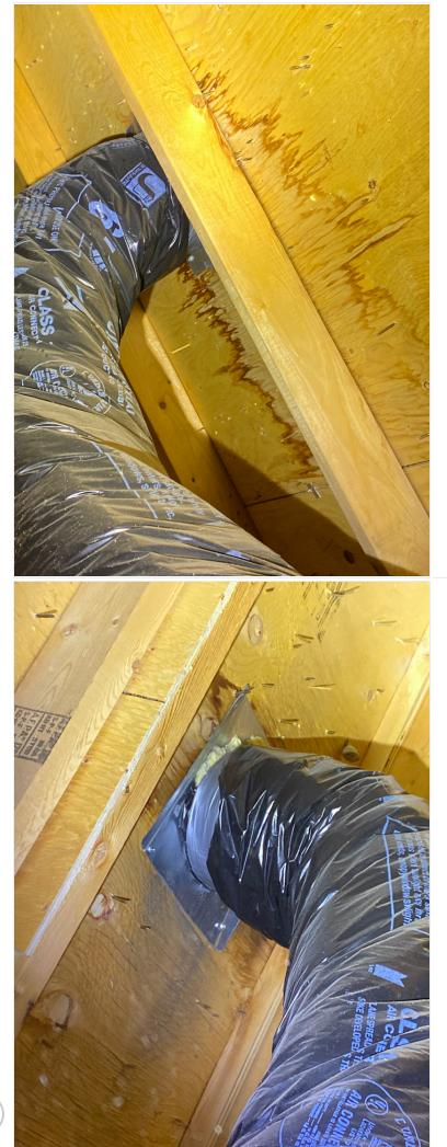
• Guest House Attic Ducts/Vents Inspected for continuous ventilation to the outside. Staining. Improve.
