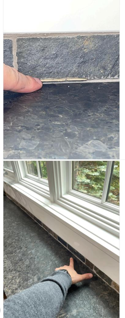
• **Grout** Generally a mixture of water, cement, & sand used to fill gaps & seal joints. Keep it clean! Depetion. Repair or Replace.
